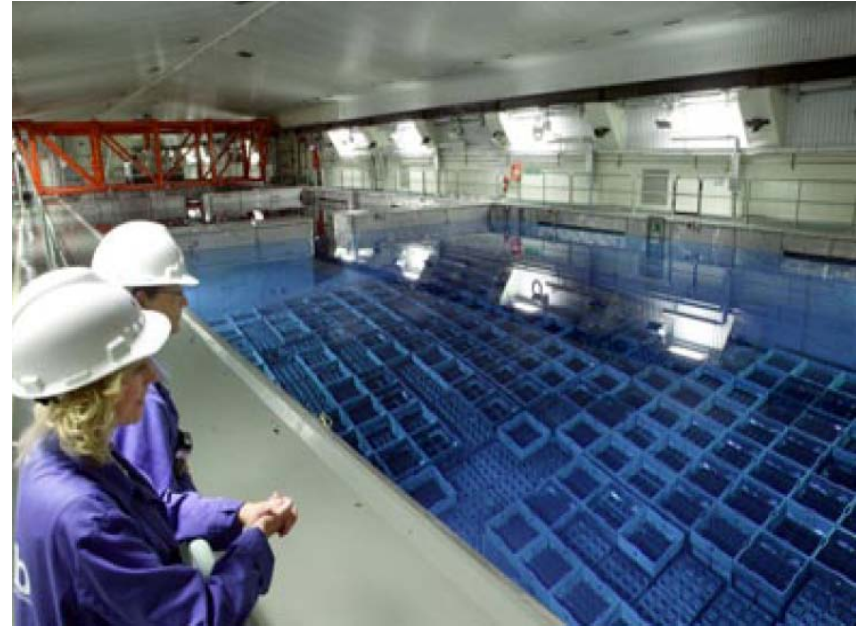
CLAB – Intermediate Storage of Spent Fuel at the Oskarshamn Nuclear Power Plant
